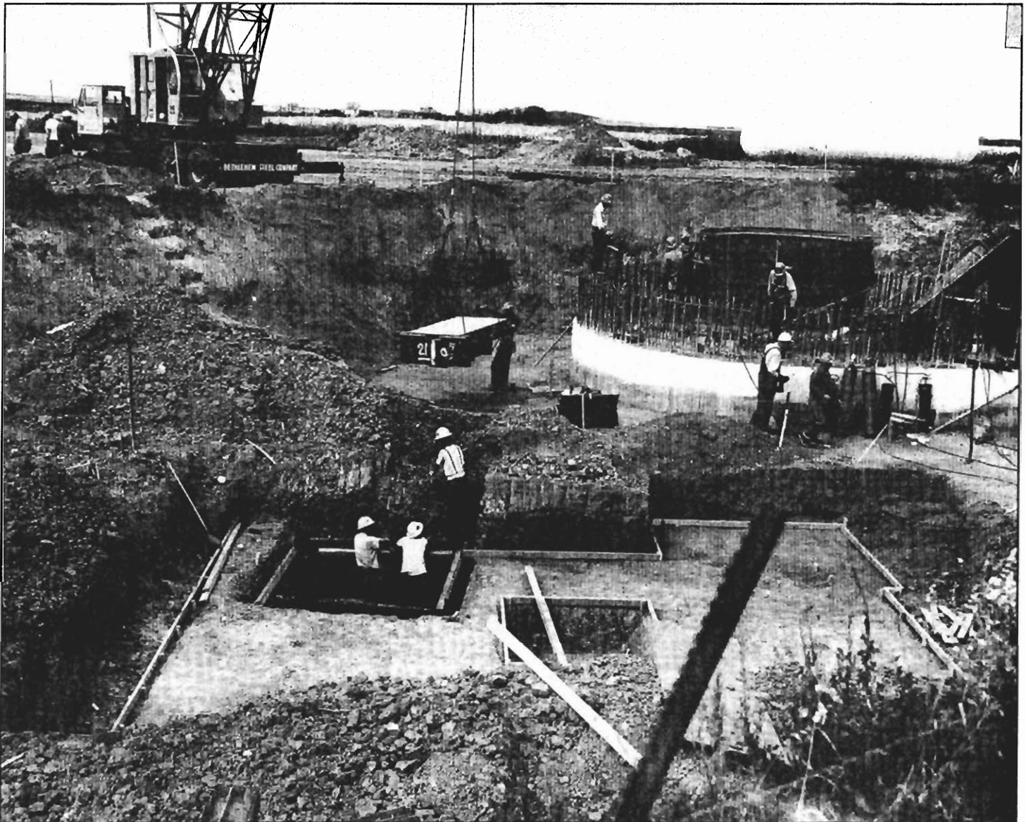
MISSILE SILO UNDER CONSTRUCTION IN 1962
