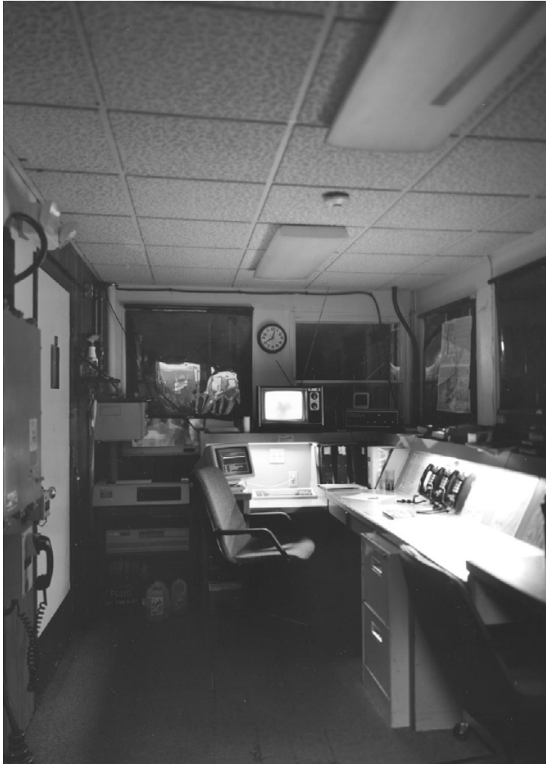
Plate 59. Delta- or Launch Control Facility, Security Control Center ( Library of Congress, Prints and Photographs Division, Historic American Engineering Record, Reproduction Number HAER SD-50-A-50 )
