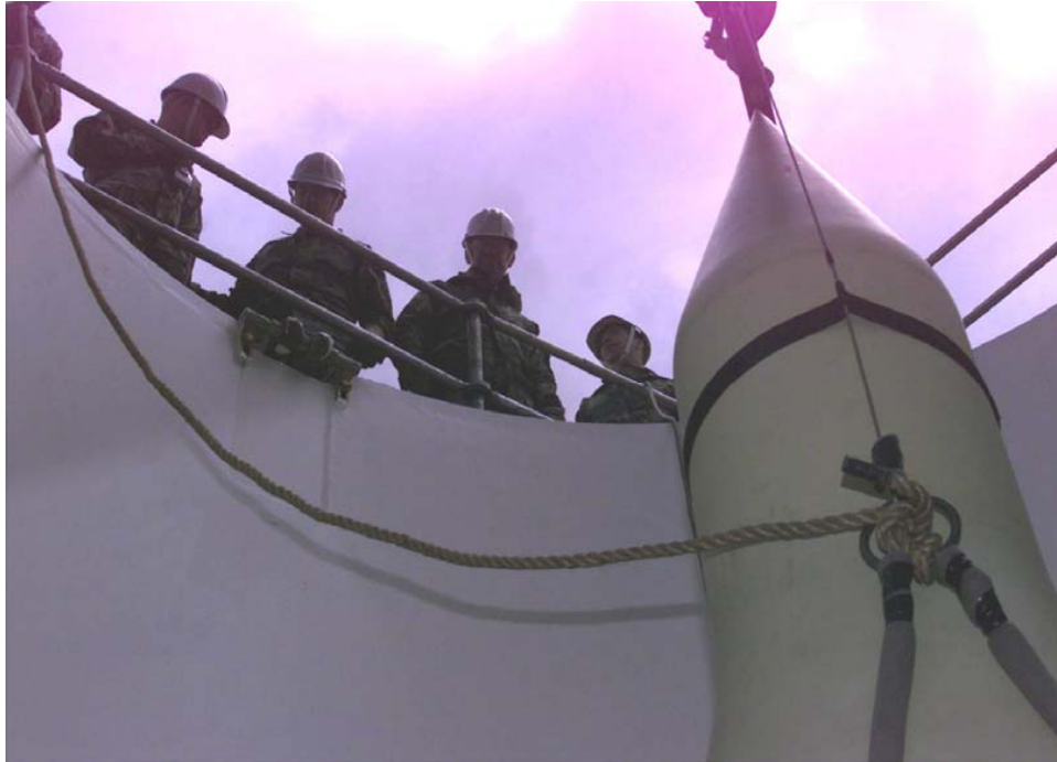
Plate 84. Training missile emplacing, Delta- 09 silo (Photograph by Staff Sergeant Melissa Phillips, F.E. Warren Air Force Base, Wyoming, U.S. Air Force photo)
