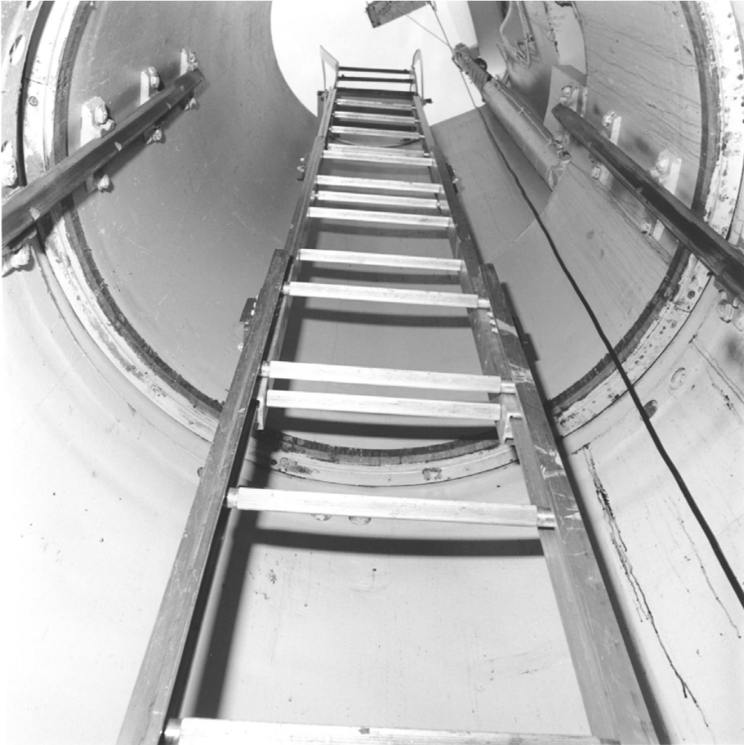
Plate 51. Personal access ladder into missile launcher, Delta-09 ( Library of Congress, Prints and Photographs Division, Historic American Engineering Record, Reproduction Number HAER SD-50-C-24 )
