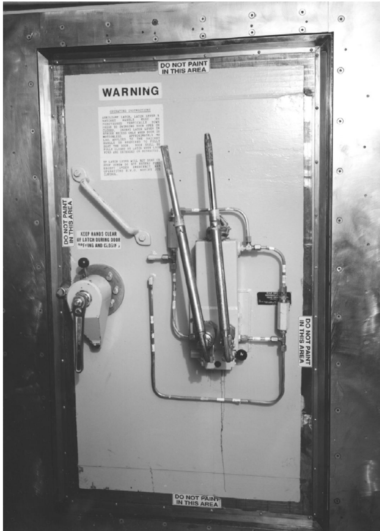
Plate 44. Interior side of blast door, Delta-01 (Library of Congress, Prints and Photographs Division, Historic American Engineering Record, Reproduction Number HAER SD-50-A-56)
