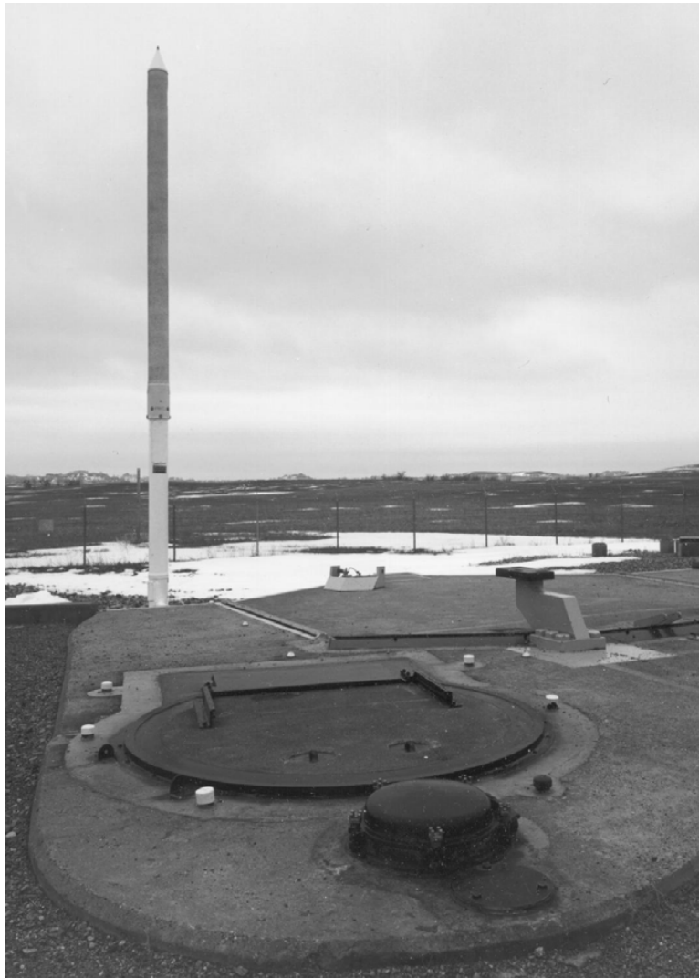
Plate 50. Topside view of Delta-09 Launch Facility with missile launcher and personnel access hatch (Photograph by National Park Service)
