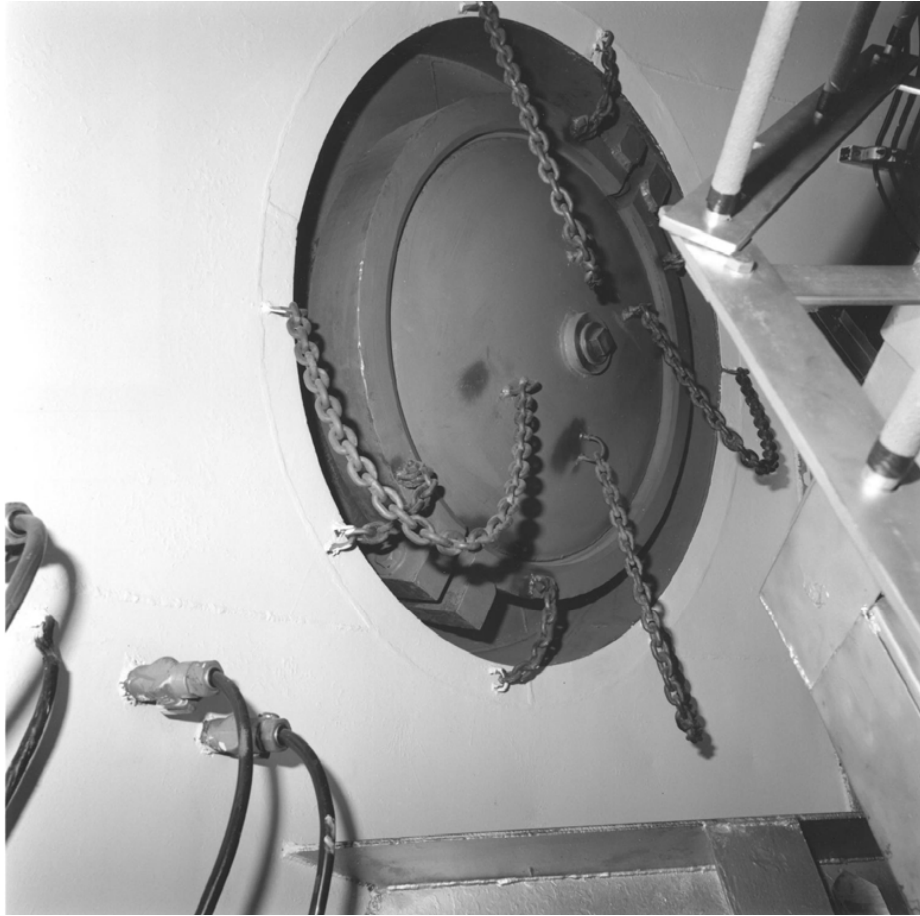
Plate 68. Launch Control Center, escape hatch ( Library of Congress, Prints and Photographs Division, Historic American Engineering Record, Reproduction Number HAER SD- 50- A- 84 )
