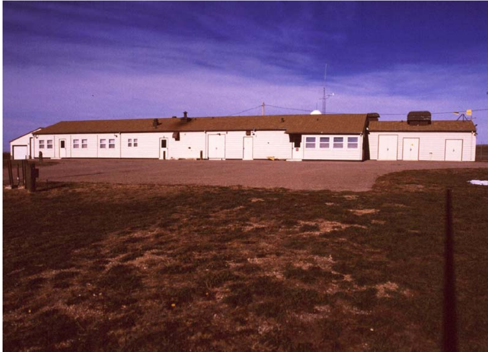
Plate 40. View of Launch Control Facility Support Building, Delta- 01 (Photograph by Mead & Hunt)
