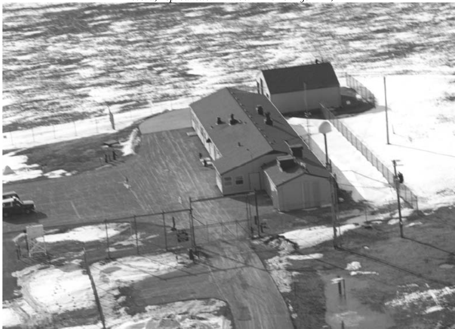
Plate 38. Aerial view of Delta- 01 highlighting the aboveground buildings used by missile crews ( Library of Congress, Prints and Photographs Division, Historic American Engineering Record, Reproduction Number HAER SD- 50- A- 1 )
