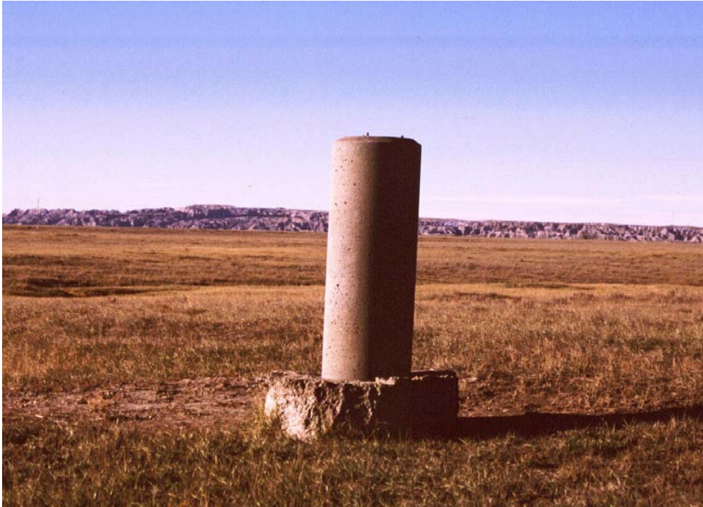
Plate 54. One of two azimuth markers located outside the Delta- 09 security fence used by guidance technicians to align the missile's guidance system (Photograph by Mead & Hunt, Inc.)
