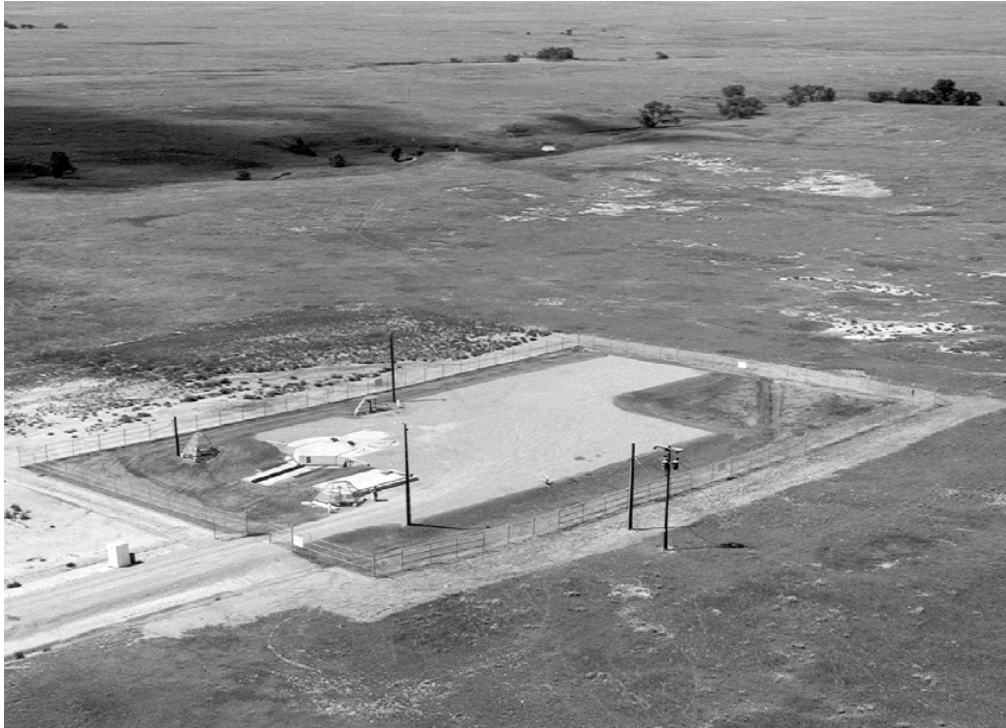
Plate 48. Aerial view of a completed Launch Facility in 1963 ( "Site Activation Chronology, Minuteman Project, Ellsworth Air Force Base, South Dakota, July 1963- October 1963," K243.012- 40, in USAF Collection, AFHRA )
