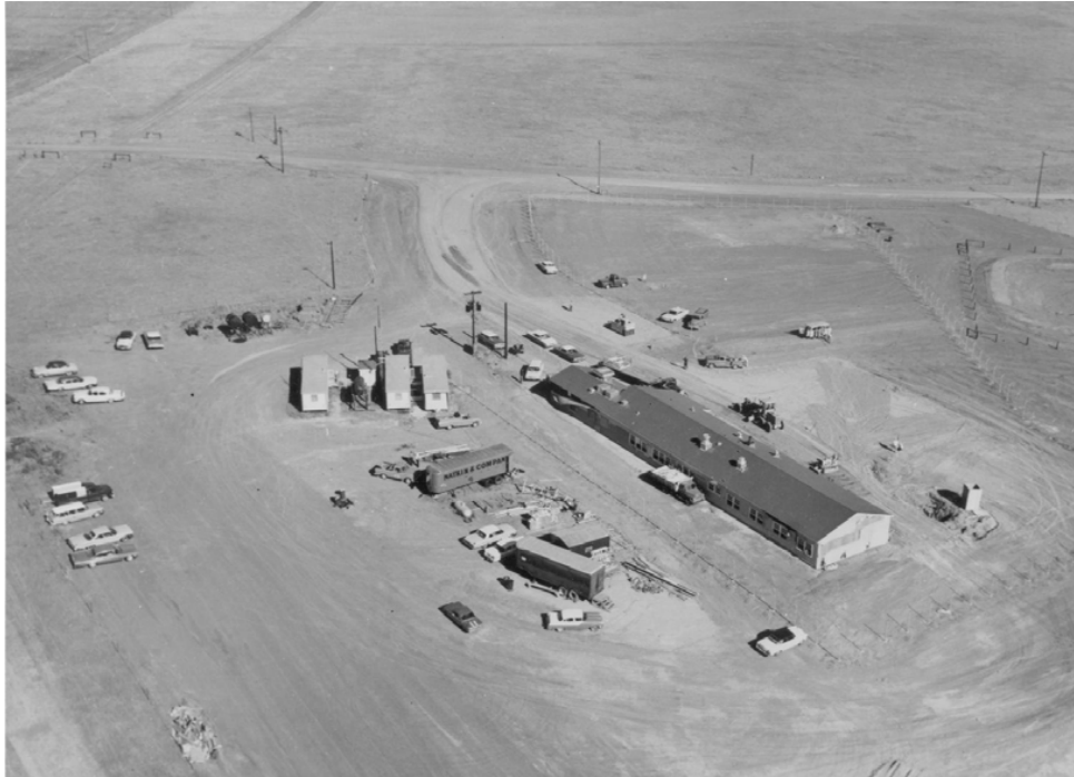
Plate 28. Aerial view of Delta-01 during construction (Courtesy of National Park Service)
