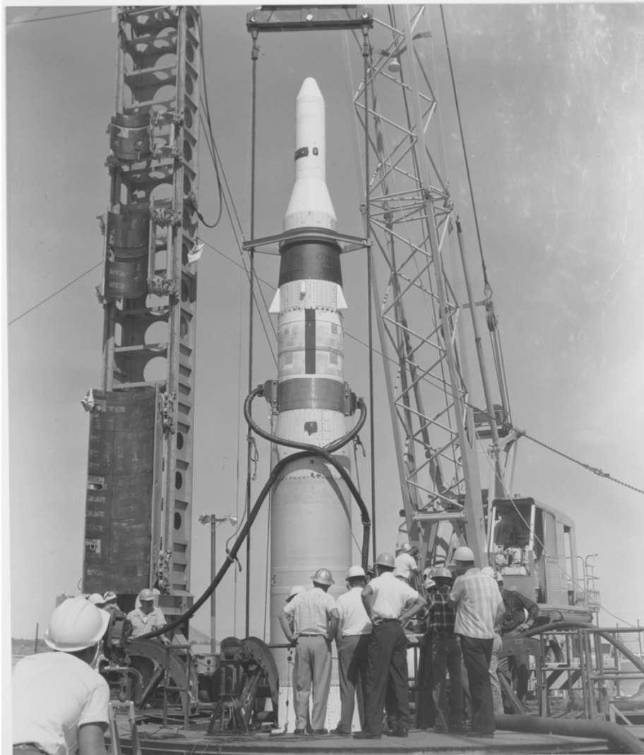
Plate II. Full-scale test of Minuteman I missile, Edwards Air Force Base, California, 1960 (Photograph No. B-08-018-1, "Guided Missiles - Boeing SM-80," U.S. Air Force Photo, Record Group 342, National Archives, College Park, Md.)
